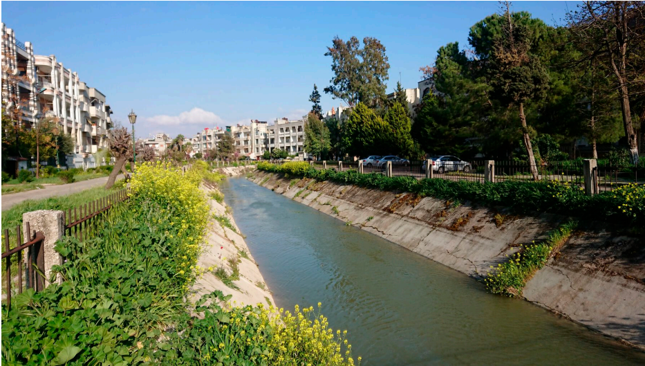
Figure 11.9a A 2021 photo of the irrigation network running through the city. Municipal decisions to let the water flow are followed by others to restrict it, an on-and-off approach not explained to the public. Image: Marwa al-Sabouni
