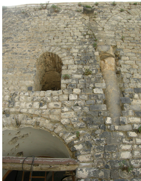
Figure 11.6a–b The war inflicted great structural damages to the mosque, revealing older pillars from a previous structure buried within its walls. These remnants might be seen as indicative a unique preservation approach that opted not to tear down, but rather to build on. Image: Marwa al-Sabouni
